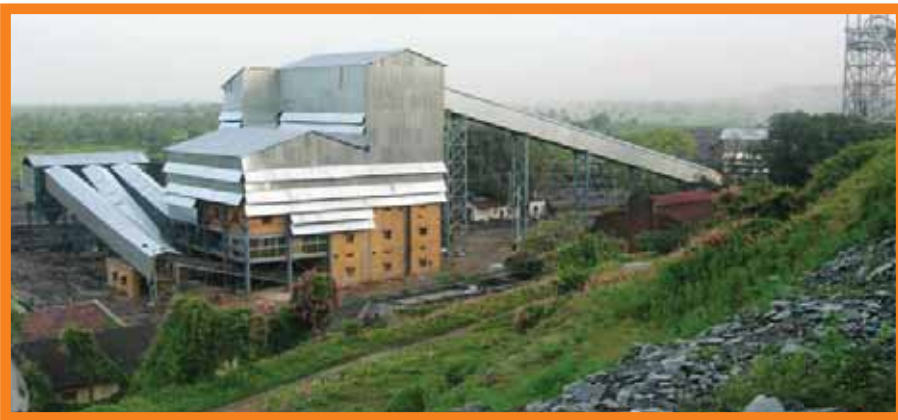
MOIL'S INTEGRATED MANGANESE BENEFICIATION PLANT OF 500000 TPA CAPACITY AT BALAGHAT
