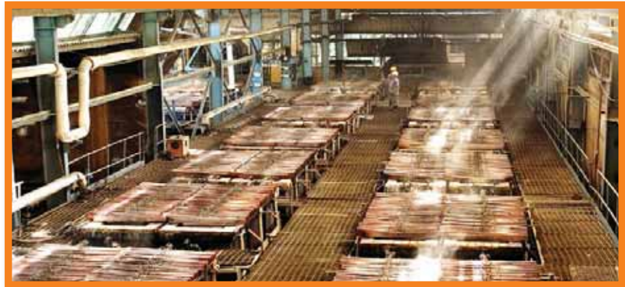
MOIL'S ELECTROLYTIC MANGANESE DIOXIDE (EMD) PLANT OF 1000 TPA CAPACITY AT DONGRI BUZURG MINE
