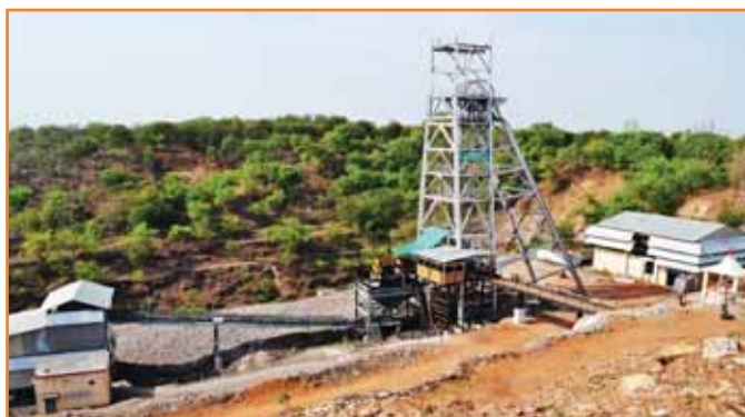
Vertical Shaft at Gumgaon Mine
