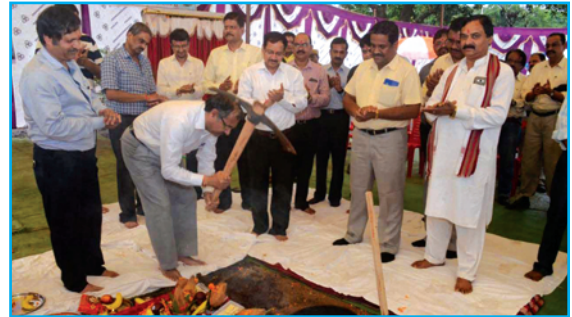
Shri M. P. Chaudhari performing Bhoomipujan of Residential Quarters at Balaghat Mine
