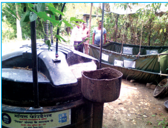
Bio Gas Unit with Vermibed Composting Unit distributed to one of the beneficiaries
