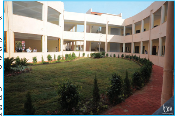
Interior view of MOIL-DAV Public School Building
