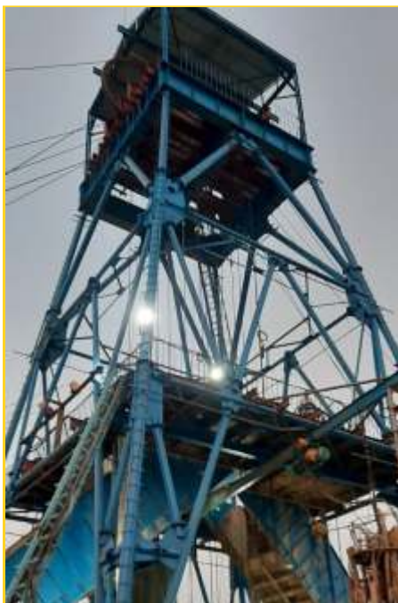
Vertical Shaft at MOIL's Mine
